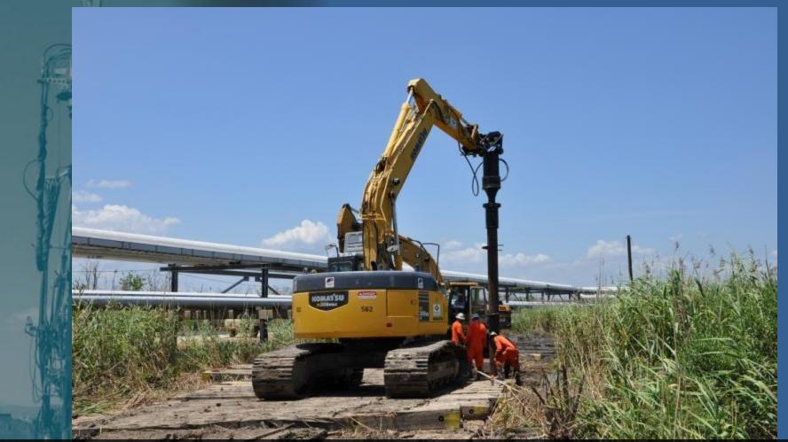
Helical pile equipment was able to access areas with soft subgrade buy using wooden mats.
