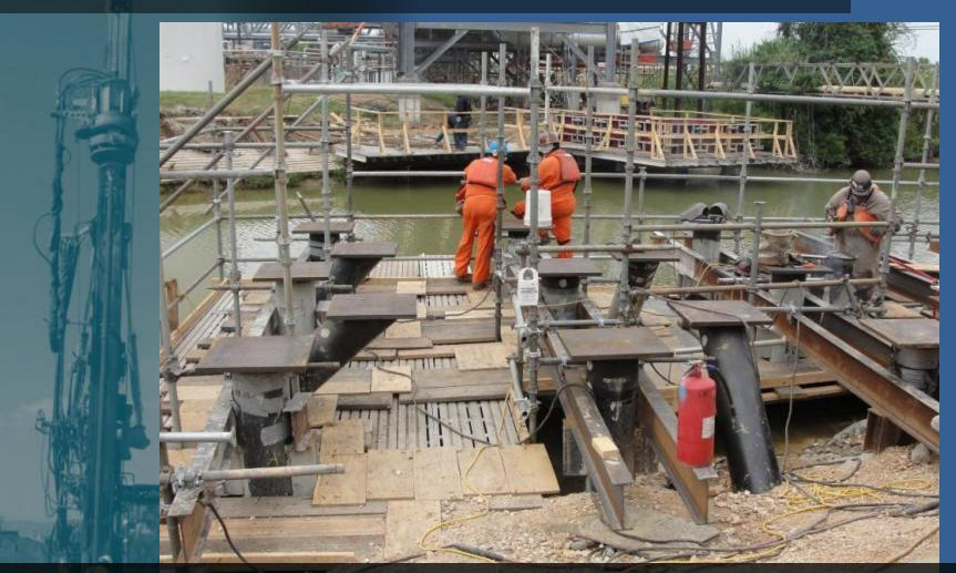
Contractor was able to replace 80 large pre-cast driven piles under this pipeline thrust block with just 20 helical piles by incorporating batter angle to handle lateral loads.
