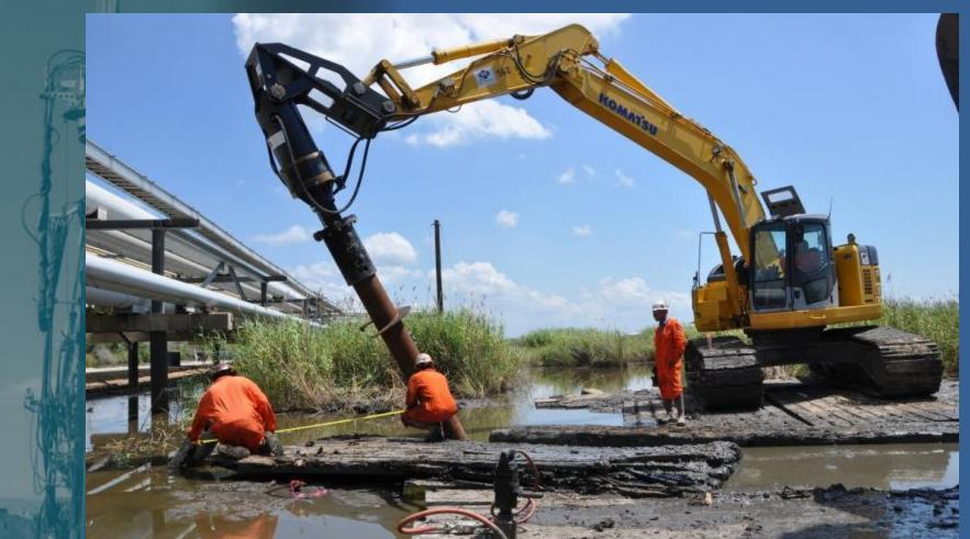
Helical piles installation equipment was able to access areas that drilling and pile driving equipment could not.
