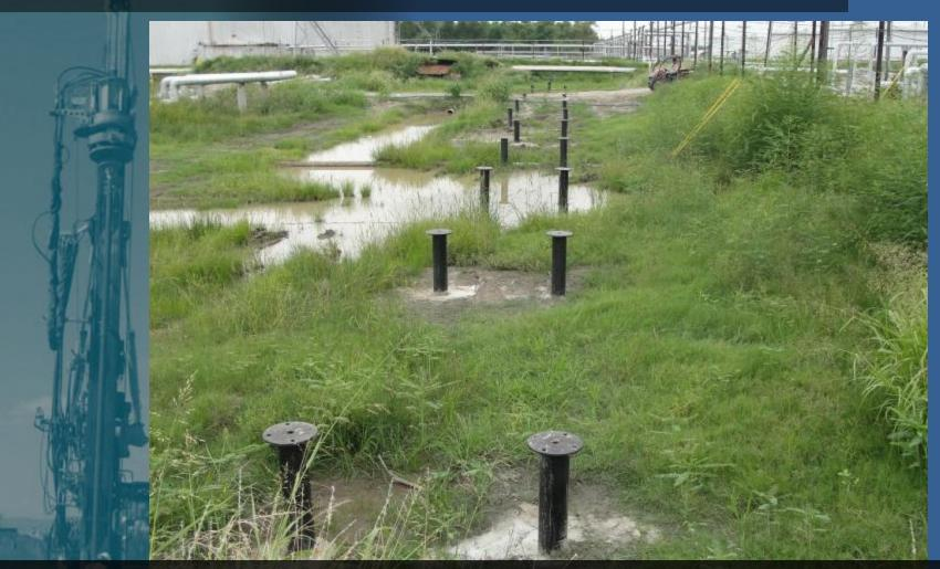
Adjustable caps were used under pipe racks so that bolting could be done instead of welding.
