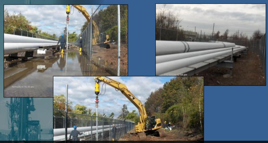
Helical piles were installed on schedule despite challenging work environment. Contractor was able to successfully and safely lift and re-align pipe lines.
